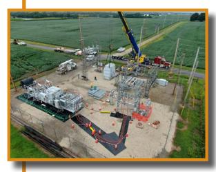
Due to the current load we carry at our Jerseyville substation, we had to bring a portable substation in to provide constant power to our Members while the work was being done. This service was provided by WVPA, free of charge. We hope to have all the work at Jerseyville completed by September 20.
