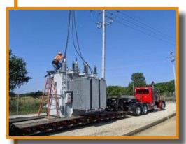
As part of our ongoing work plan, we utilize a dissolved gas analysis program to analyze oil samples from the substation transformers. This analysis gives us a method for rating the transformers performance and life expectancy. Based on that work we determined that the transformers at Jerseyville and Bunker Hill were near the end of their useful lives and would need to be replaced or reconditioned.
