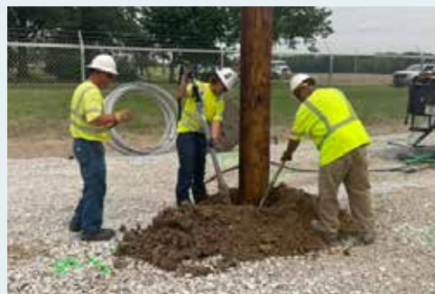
Installing pole outside of substation.
