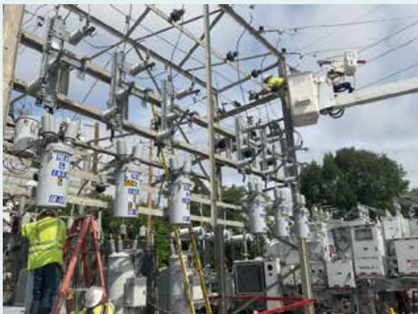
Disconnecting components for mobile sub installation.
